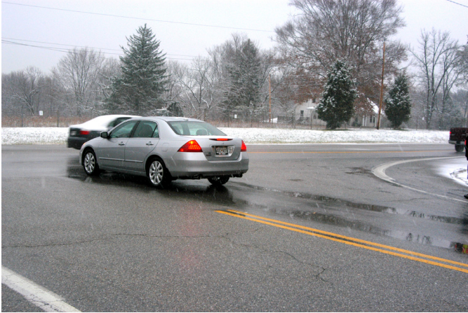
Water ponding in wheel ruts.
