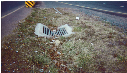
V-shaped grate in median.
