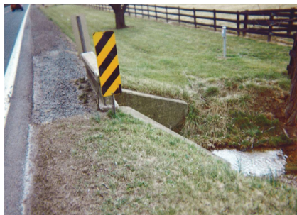
Rigid headwall delineated with Type 3 Object Marker.
